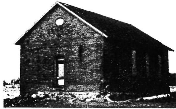
45006 The Schrock School replaced an earlier frame school and closed its doors to students in 1924.
